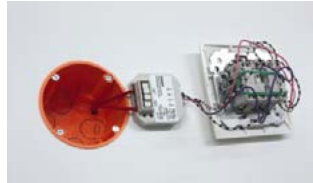
01 Connect DALI and switch in the flush-mounted box
